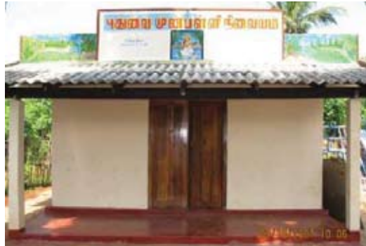
The recently renovated pre-school building
